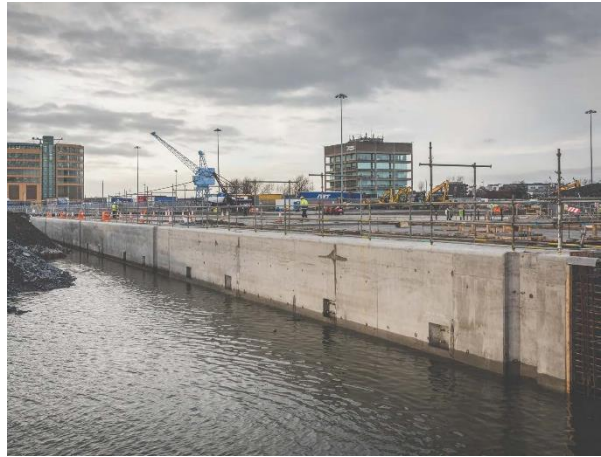
(b) Quay wall for harbour infrastructure (Image source: Roadbridge ltd)
