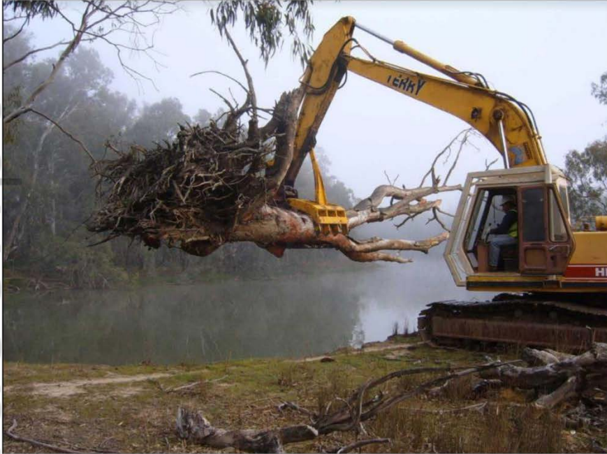
Figure 6. Placing a large log into the Murray River as part of the Murray Darling Basin Authority's Living Murray Program (photo courtesy of Jarod Lyon).
