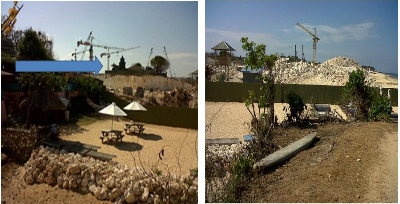
Figure 3.5 These images show the cut and fill activities, the proximity of the project to the local temple (marked with a blue arrow), the huge stack of limestone, and the installation of a zinc fence around the Mulia Project. Source: WALHI Bali.
